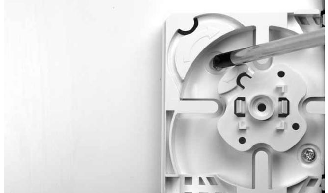
2.3 Secure the box onto the wall (optional).
